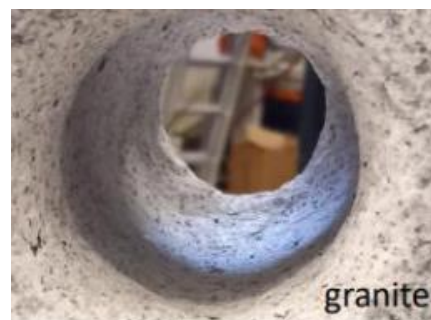
Thermally spalled borehole
